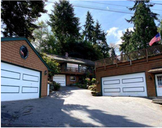
Plate 1. Existing house with detached garages, looking south.
